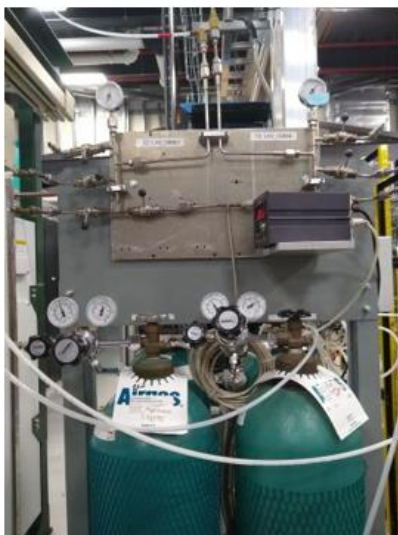
Large Gas Cylinders and Main Manifold
